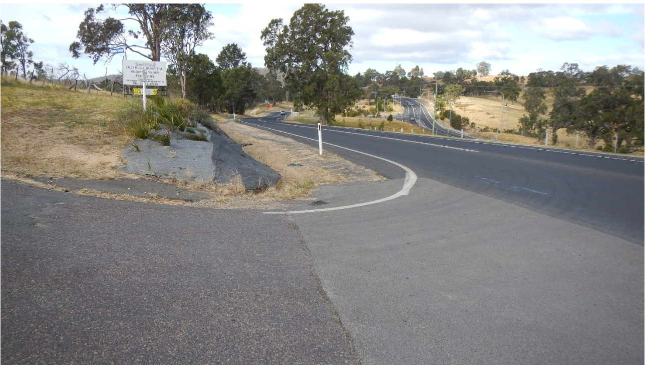
Figure 4 Intersection looking south with ample sight distance
