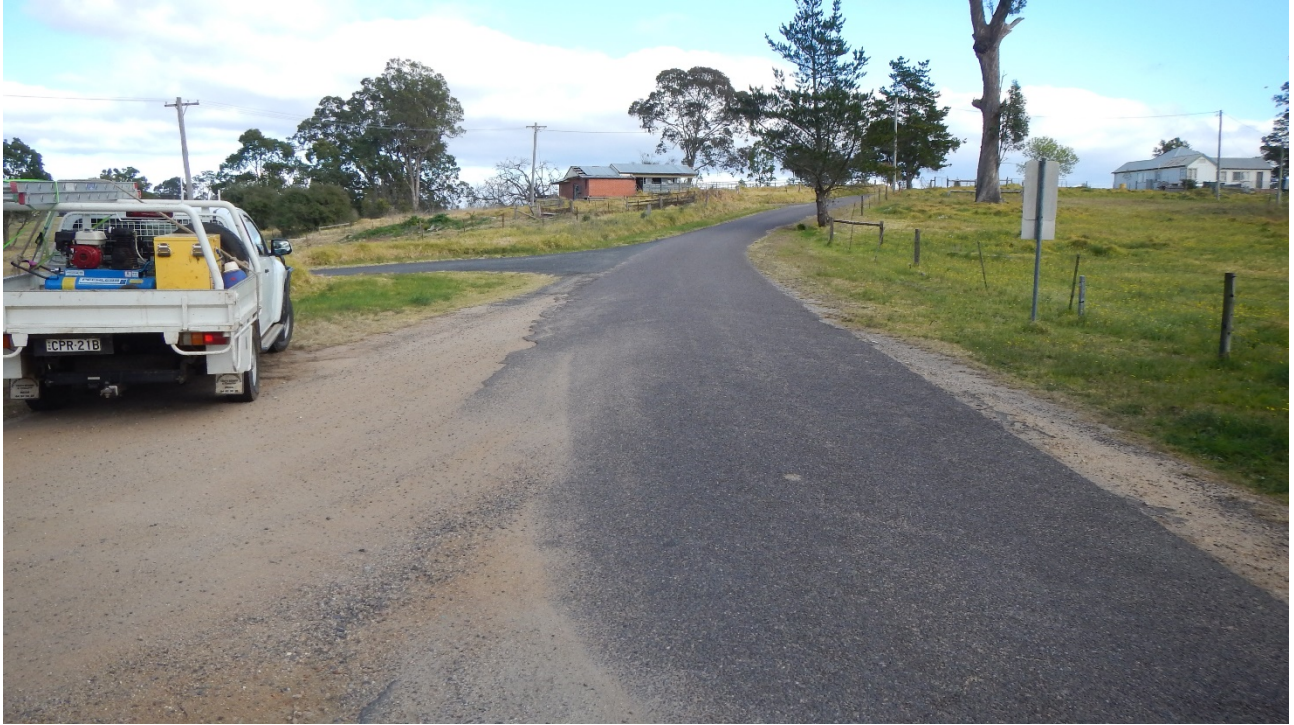
Figure 2 existing access road (Corkhill St) with 4 wide seal and passing shoulders
