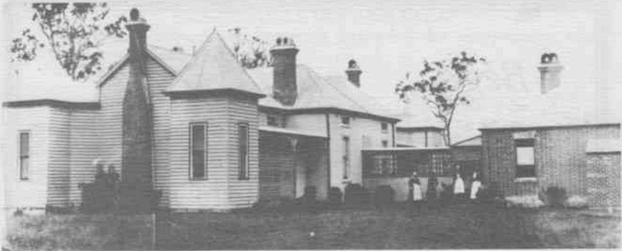
Rear view of the original hospital, built 1889
