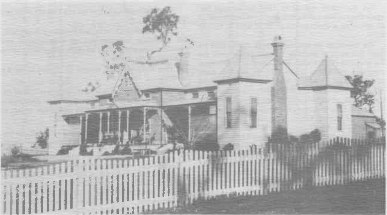
The original hospital building
